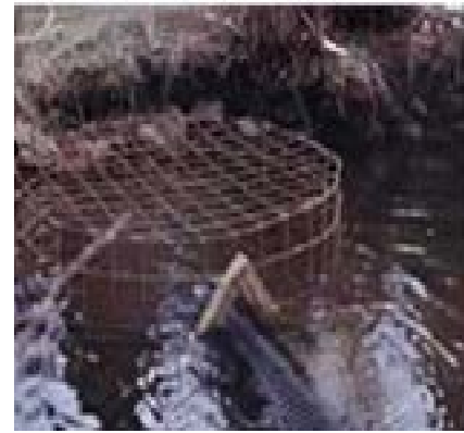
(Above) Inserting a flow regulator into a dam to control the pond water level.
